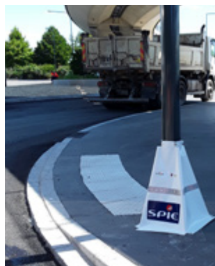
Protection chantier poteaux
