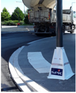
Protection chantier poteaux
