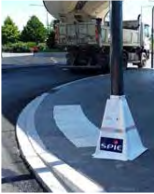
Protection chantier poteaux
